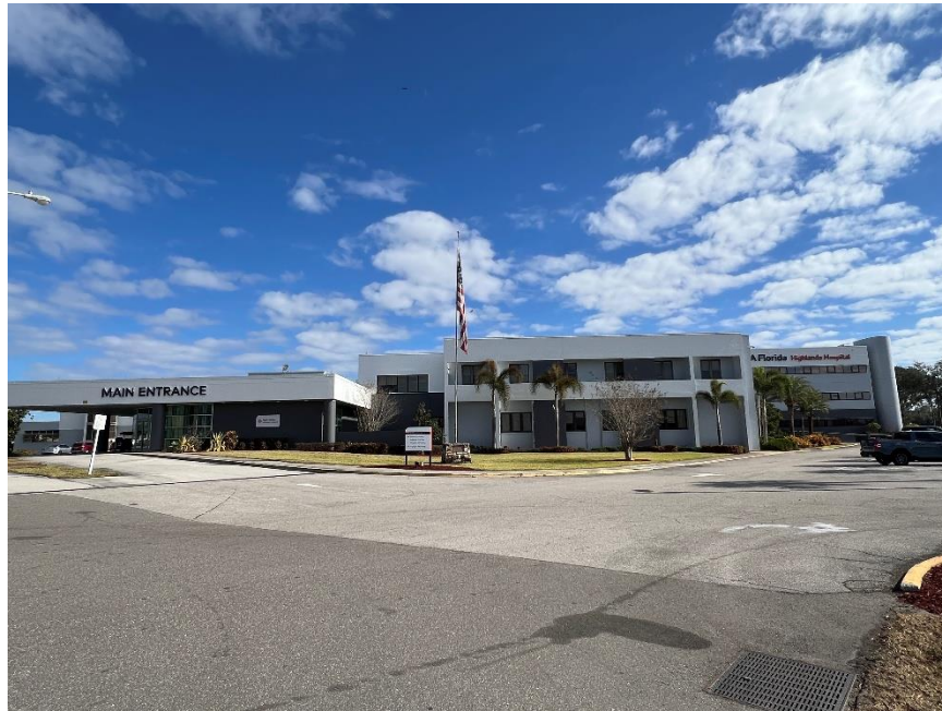
Hospital Front Exterior
